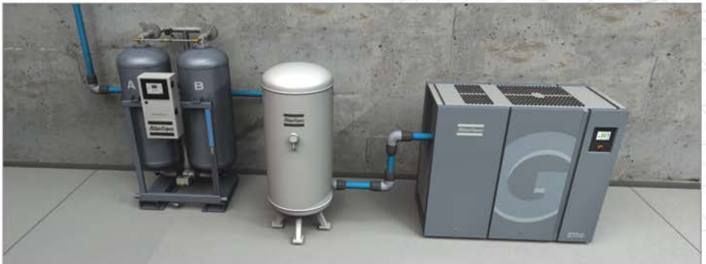
CD dryer installed with reversed piping option.
